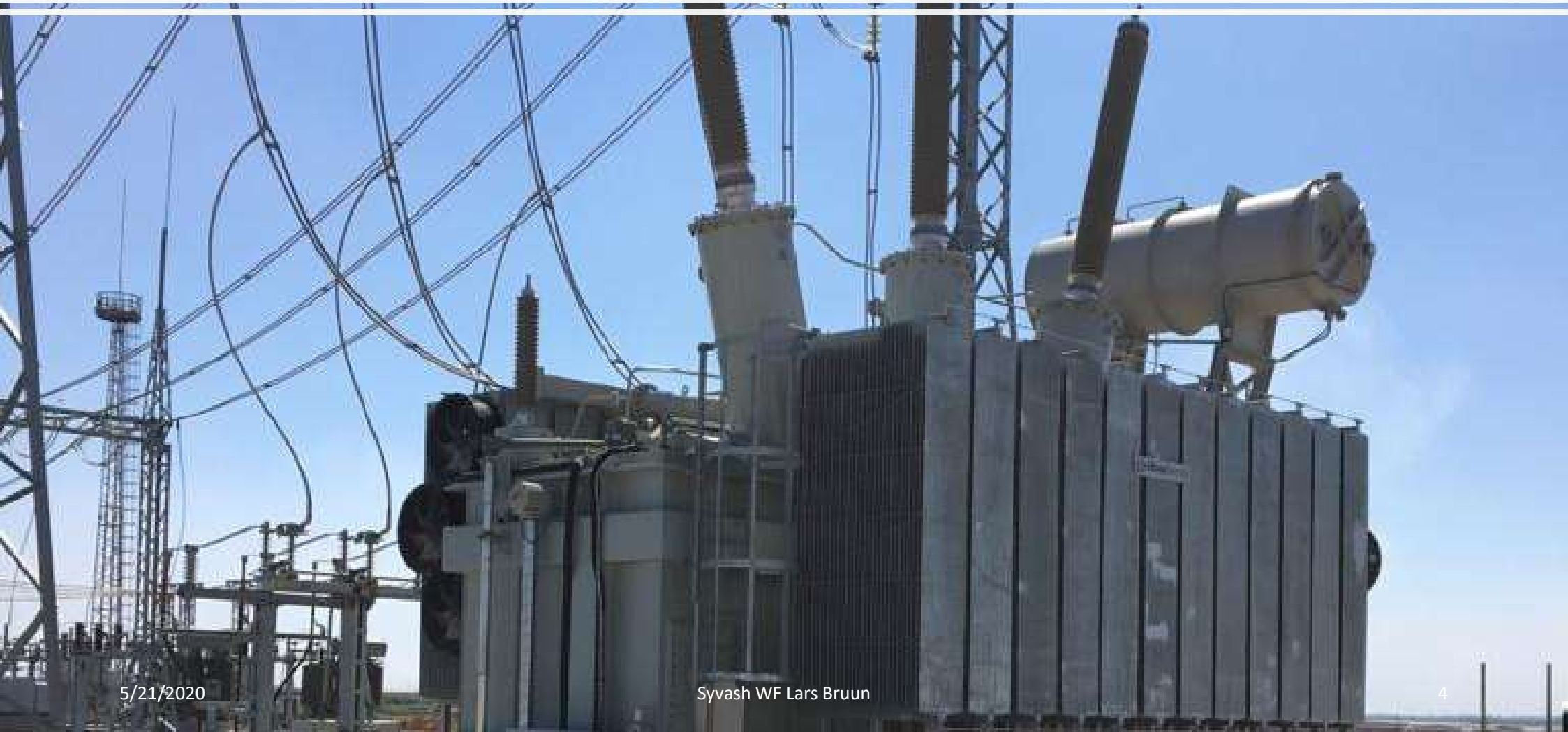
Syvash Substation 1 st main transformer (one of two)
